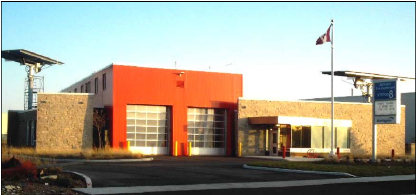
Burlington Station 8 (picture courtesy of Rob Simpson)
