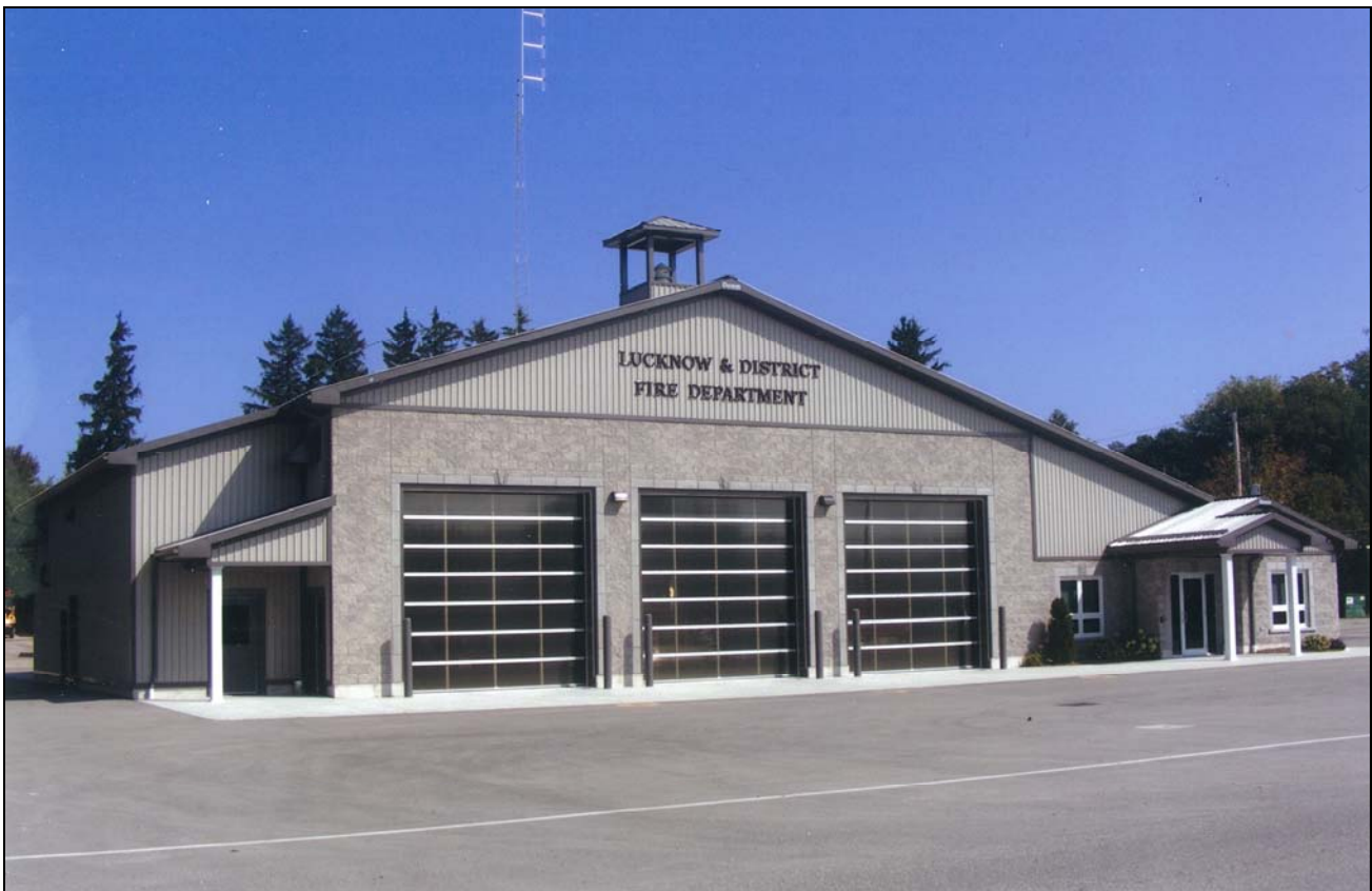
Lucknow Fire Hall, also in Bruce County, is home to a pumper, two tankers and a rescue. Built in 2010, it's located at 725 Campbell St. (Neil McCarten photos).
